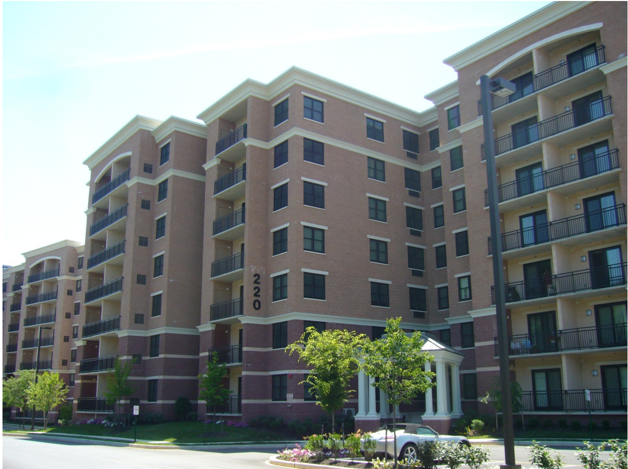
Figure 1: North-west view of Tower 'B', showing canopy entrance.
